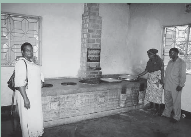
The new energy saving stove in a spotless school kitchen. Photo ©: Sustainable Moshi Project
